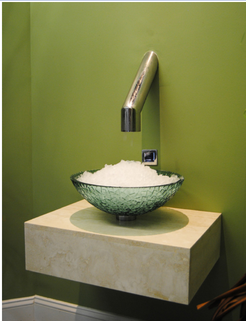
Sensor-activated Ice Fountain with distinct glass dish and positioned near a thermal room
