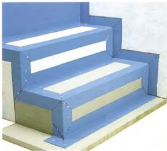
a) Installation of compound sheetings
