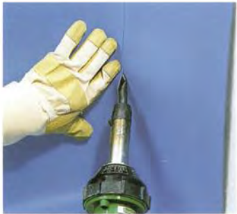
p) Welding of corner seam
