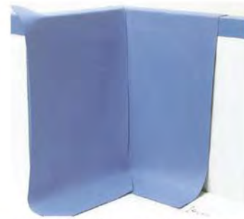
o) Condition after cut to size of corner
