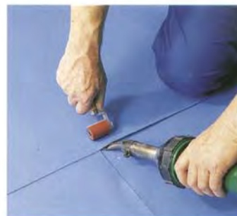
c) Subsequent pressing with roller for fixing a T-joint
