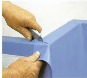
q) Cutting at the top corner outside
