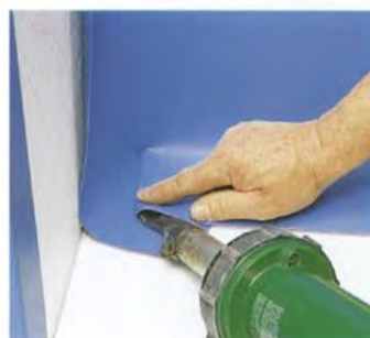
l) Welding of the loop outside
