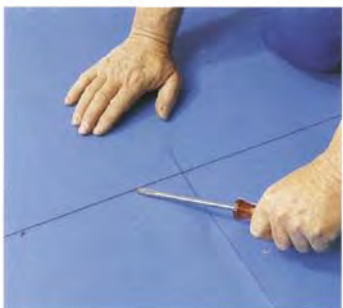
d) Seam inspection
