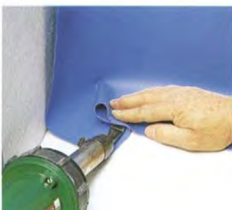
k) Welding of the loop inside
