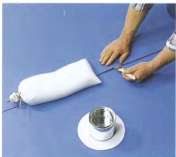
a) Welding with welding agent
