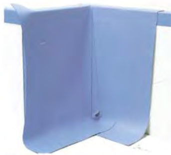
n) Marking of corner seam
