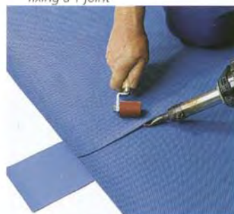
f) Welding of NGP
