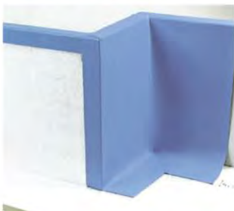
s) Outside corner after welding
