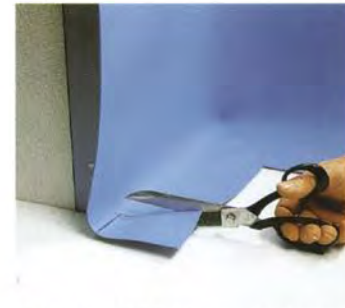
r) Cutting at the bottom corner outside
