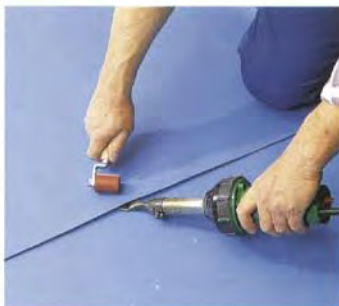
b) Hot gas welding
