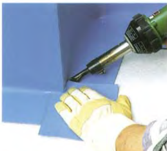
v) Welding of corner part
