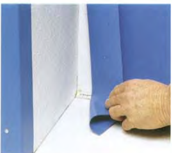
j) Corner under prestress on the backside
