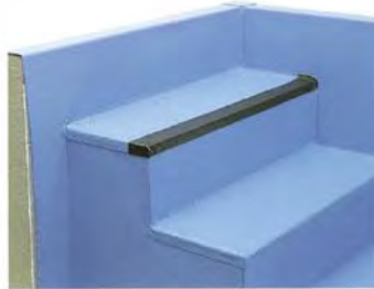
e) Nosing of stairs in contrasting colour
