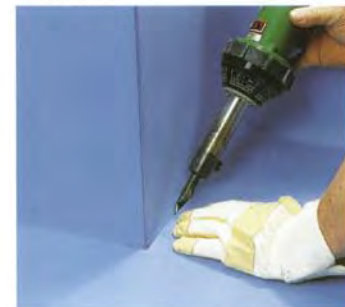
x) Connection of floor lining
