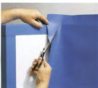
h) Cutting at the top corner inside
